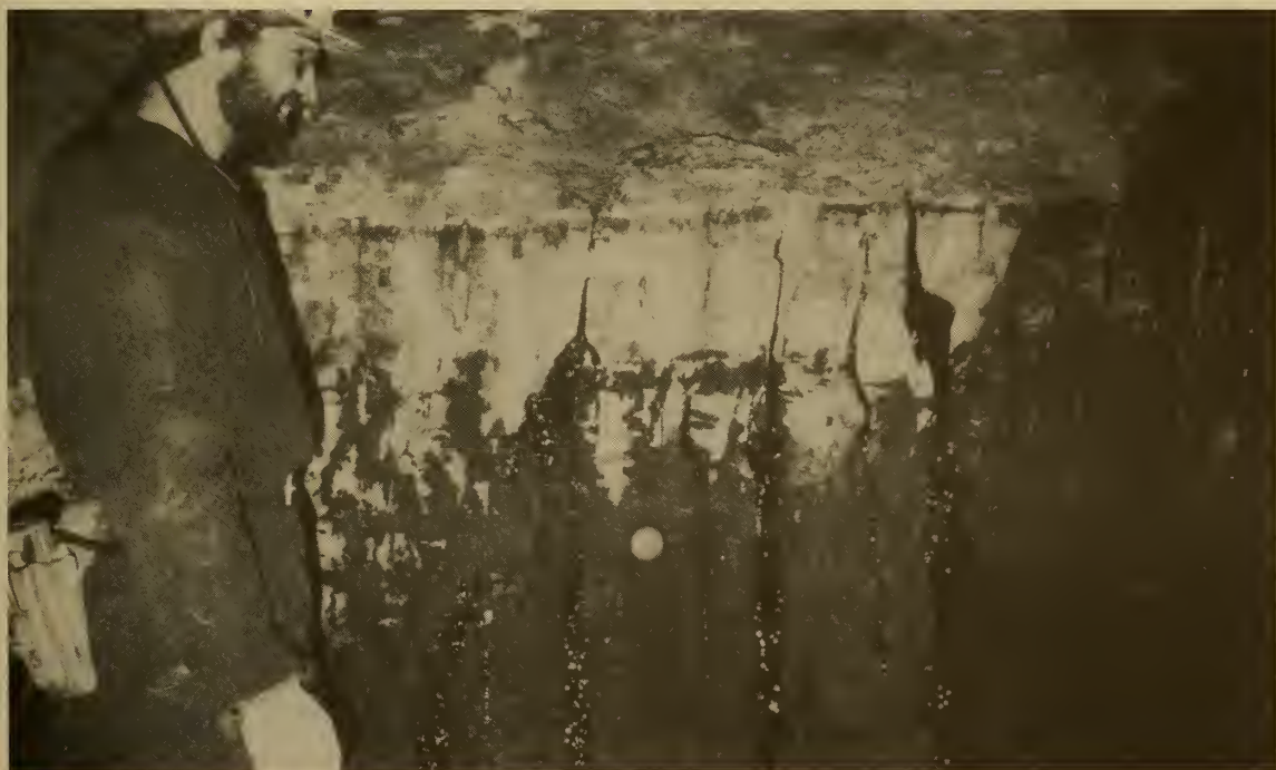
FIGURE A-8. - Polyurethane grout emerging from strata.
