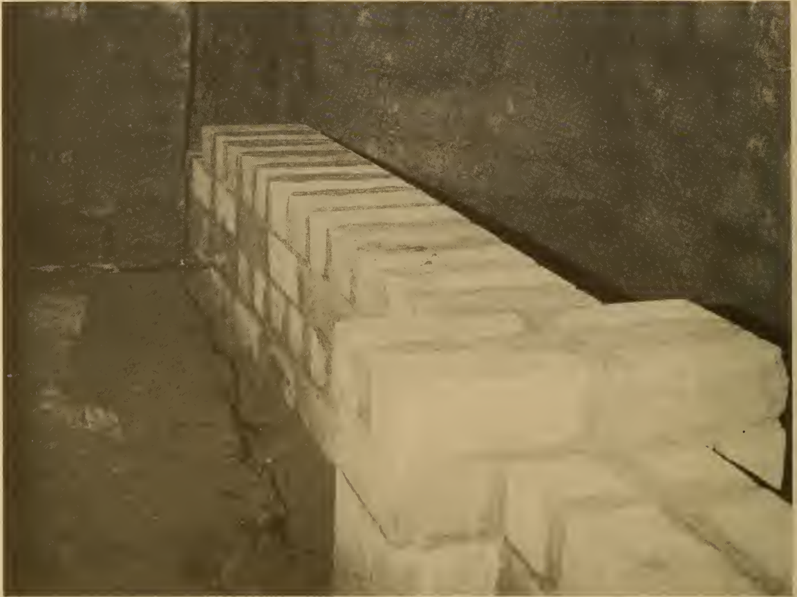
FIGURE A-3. - Bulkhead under construction in Safety Research Coal Mine.
