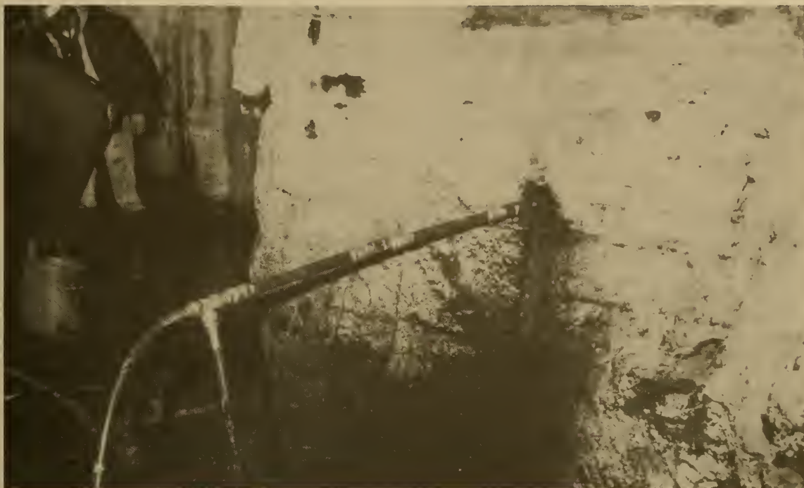
FIGURE A-7. - Packer-mixer assembly installed in borehole.
